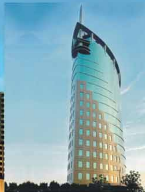
Gateway Tower, Gurgaon
