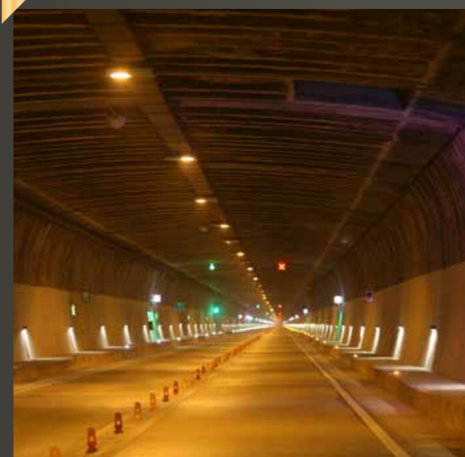
CHENANI-NASHRI TUNNEL, JAMMU & KASHMIR
