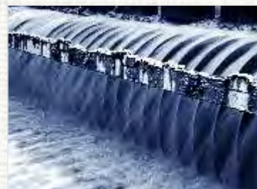
Sewage treatment plant and clean water plant
