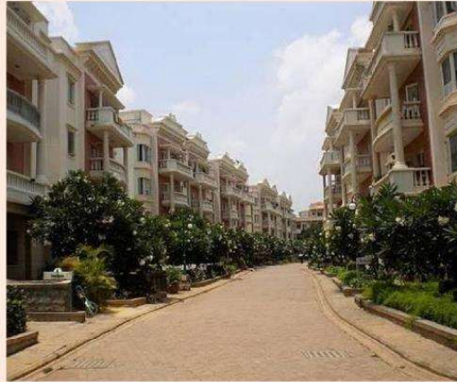
TATA Sherwood, HAL 376 Delivered Homes
