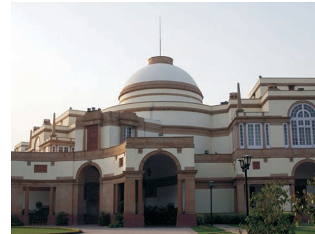
Hyderabad House - New Delhi, built by late Khan Bahadur Abdul Karim Babukhan for the Nizam of Hyderabad
